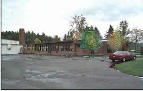
Renovation of Five Schools Fort Lewis/McChord AFB
