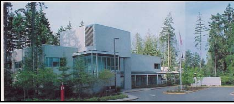
Regional Operations Center Submarine Base Bangor
