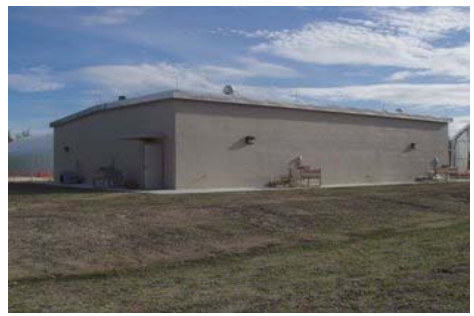
Remote Switch Facility Navy, Diego Garcia
