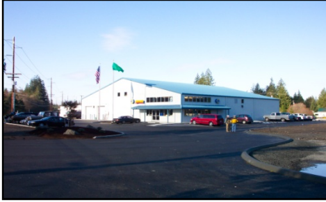
NAPA Retail Store/Warehouse Port Hadlock, WA
