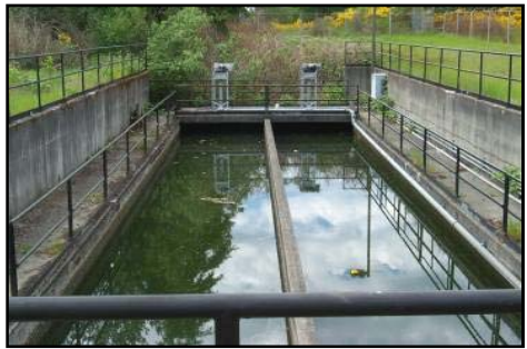
Stormwater Outfall 7 Fort Lewis
