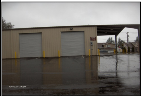
City of Bremerton Fire Department Storage Building
