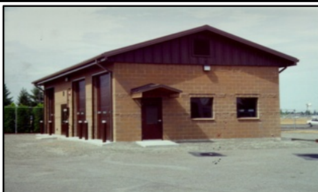
Hazardous Waste Transportation Facility McChord AFB
