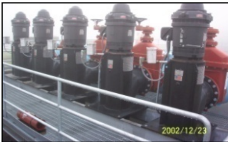
Stormwater Outfall 2 Fort Lewis
