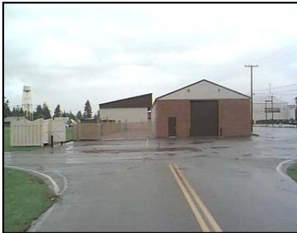
Building 1218 Alterations McChord AFB
