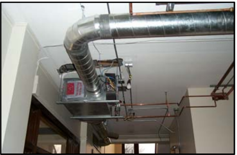
State of Washington Newhouse Building HVAC Upgrades
