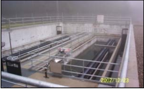
Stormwater Outfall 3 Fort Lewis
