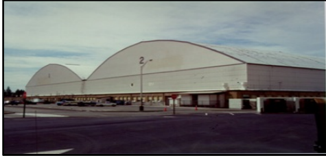
Alter Hangar 1 and 2 Side Shop Structures McChord AFB
