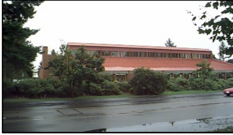
Grandstaff Library Roof Replacement Fort Lewis
